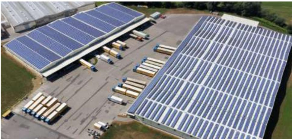
**Figure 11: Example of good and non-optimal integration of PV on the building's roof**
