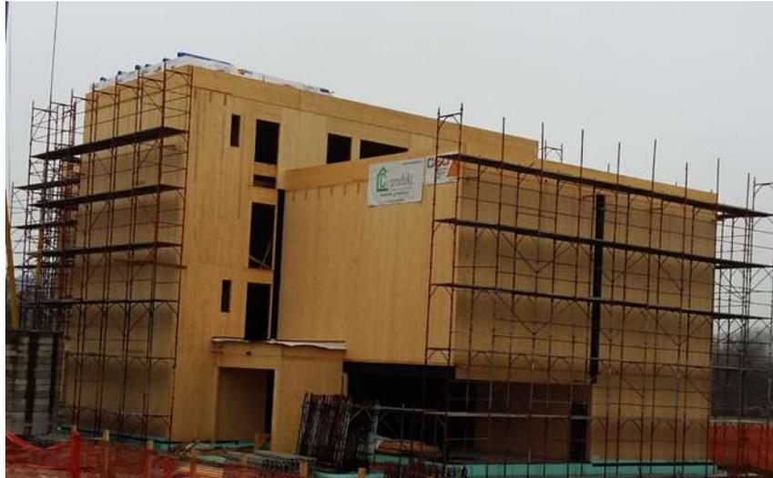
**Figure 12: Example of a Squash hall, with wood as the basic construction material**
